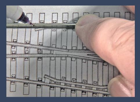
Figure 41: I take a piece of code 83 rail, lay it against the guard rail area of the turnout template, and mark the length with a Sharpie®.
