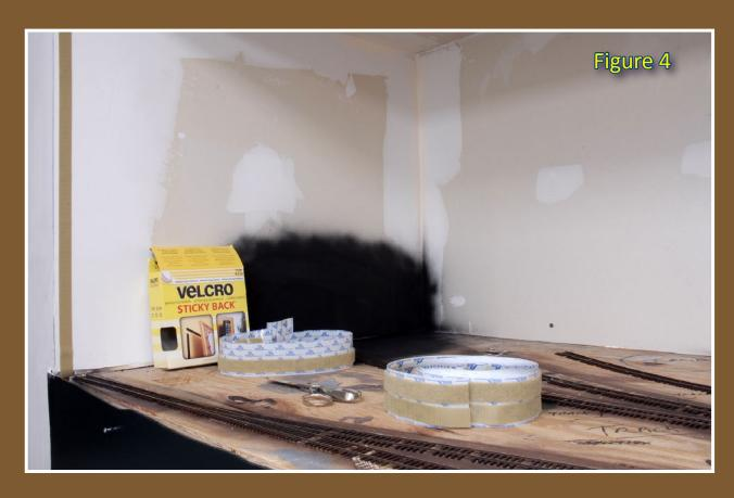
Figure 4: To secure the polystyrene backdrop, I used strips of Velcro. This is much neater and cleaner than using adhesive, and it gives me the flexibility of removing it at a later date if changes need to be made.
