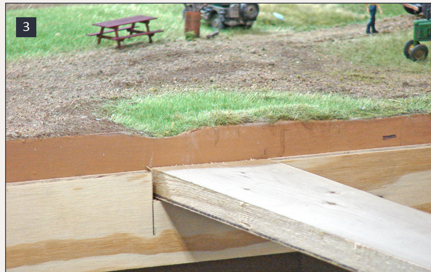
3: Adding notches into the plywood frame to hold the 1x4 support stringers.
