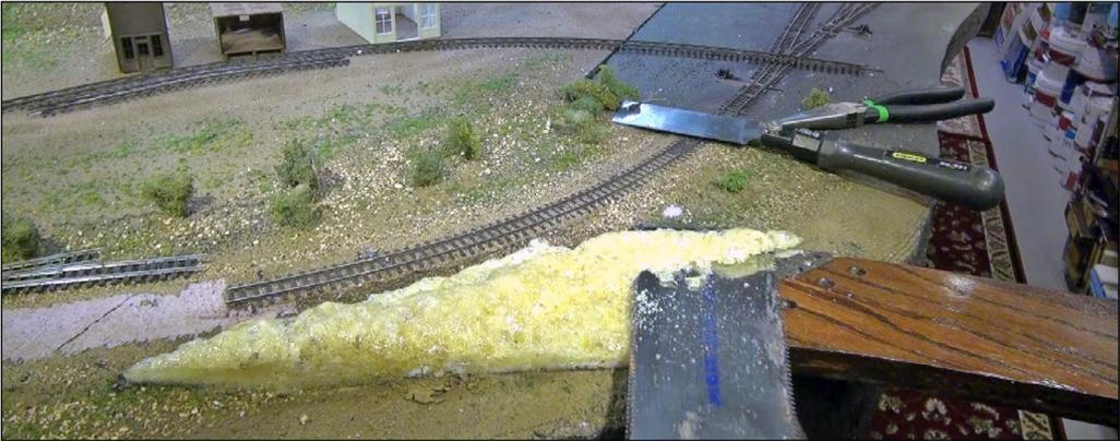
24. To build up the approach to make a smooth transition from the Blackstone II layout to the lift-out plywood, I built a dam from styrene and filled this area with a layer of Gorilla Glue, thinking this would expand into road bed. It did! Another new idea! I cut it smooth with a saw, making a solid base for laying track.
