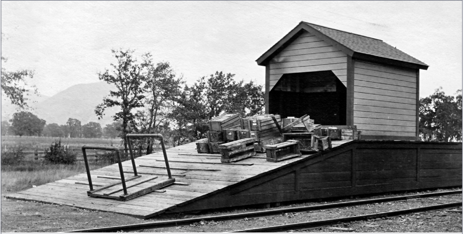
8. The freight shelter at Los Guilicos, California, north of Kenwood on the Santa Rosa Branch, in a 1912 photo from Bender's book. This 10 x 12-foot shed stood on a 16 x 20-foot platform, not counting the ramp. SP photo, Shasta Division Archives
