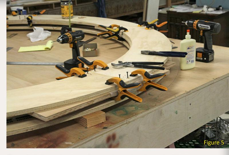
Figure 5: I clamped a piece of scrap plywood under each of the joints in the second lap roadbed to "splint" the freshly biscuited joint. The track on the first (lower) lap roadbed made simply clamping the two laps together a poor choice. Using the scrap keeps the joints nice and flat.
