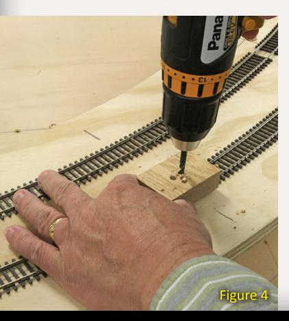
I also soldered 22-gauge solid track feeder wires to the rails at this time, bringing them out to the edges of the helix roadbed where they'll connect to 12-gauge stranded bus wires.
