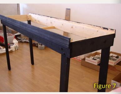
Figure 7: The final step in building the basic cradle is painting it.
