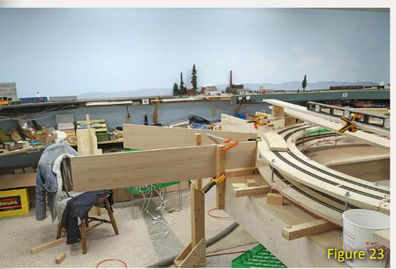
Figure 22: I decided to screw and glue 2x2 cleats to the helix table side plates to hold the joists. Doing this with a two-man crew avoided a lot of crawling back-and-forth since the screws needed to go through the side plates and into the cleats for maximum strength.
