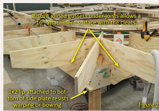
Figure 25: TROUBLE! After Mike and Joe left I discovered that the joists were alarmingly flexible when attached only to the 8" of the cleats that protruded above the helix table surface. The solution was obvious – I added gusset plates under the table-end of the joists.
