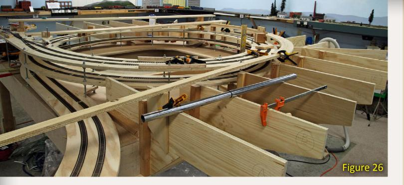
where an under-the-table joist was located, it was very stiff. Otherwise the side plate deformed, letting the end of the joist move up and down. We addressed this problem by screwing and gluing a 1x2 "lip" at the bottom of the side plate turning it into an L-girder (figure 25). Now the joists were stiff! I beveled the ends of the joists for better access to the area underneath them.
