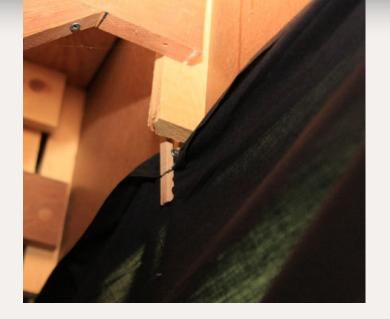
Figure 5: Spring-loaded clothes pins make curtain installation and removal easy.
