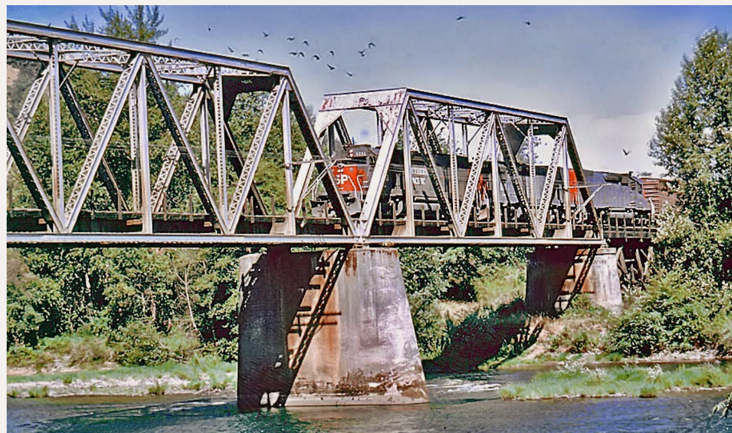
Figure 4: To carry code lines across a stream, the Southern Pacific attached crossarms to the sides of this bridge over the Umpqua River in southern Oregon. Joe Fugate photo.
