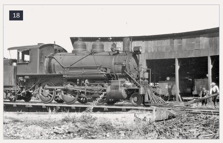
18: In this photo, the crew is turning the No. 28 on the turntable at Merced, probably around 1944 or so. But, what was also of interest to me is the pile of "junk" in the bottom right corner of the photo. The large wooden object is a sawhorse, not your typical carpenter sawhorse but a heavy-duty one. There are also some springs, most likely from freight car trucks, and a lot of scrap material. This pile of "stuff" shows up in some other prototype photos of the area. – *Photo by Stanley Snook*
