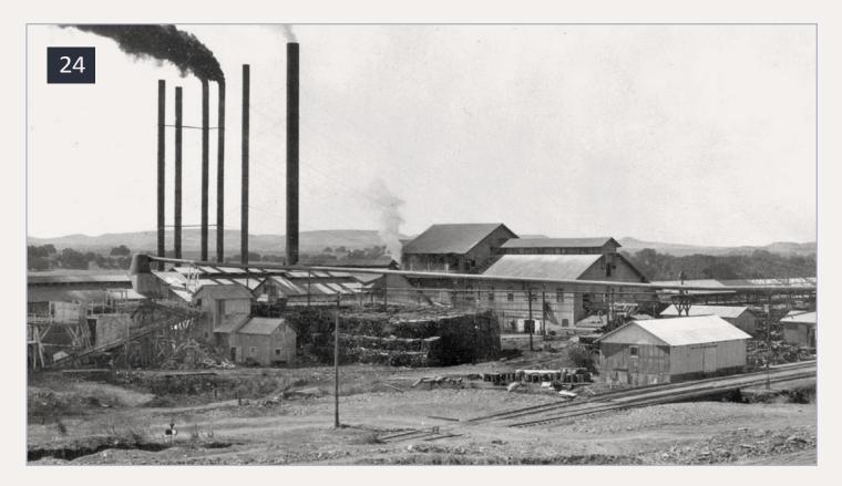
24: There was a very large lumber mill at Merced Falls which was served by the YV. The multiple smoke stacks mark the location of the boiler house while the two large buildings in the middle of the photo comprise the saw mill. The building along the track was the Electrical Shop.
