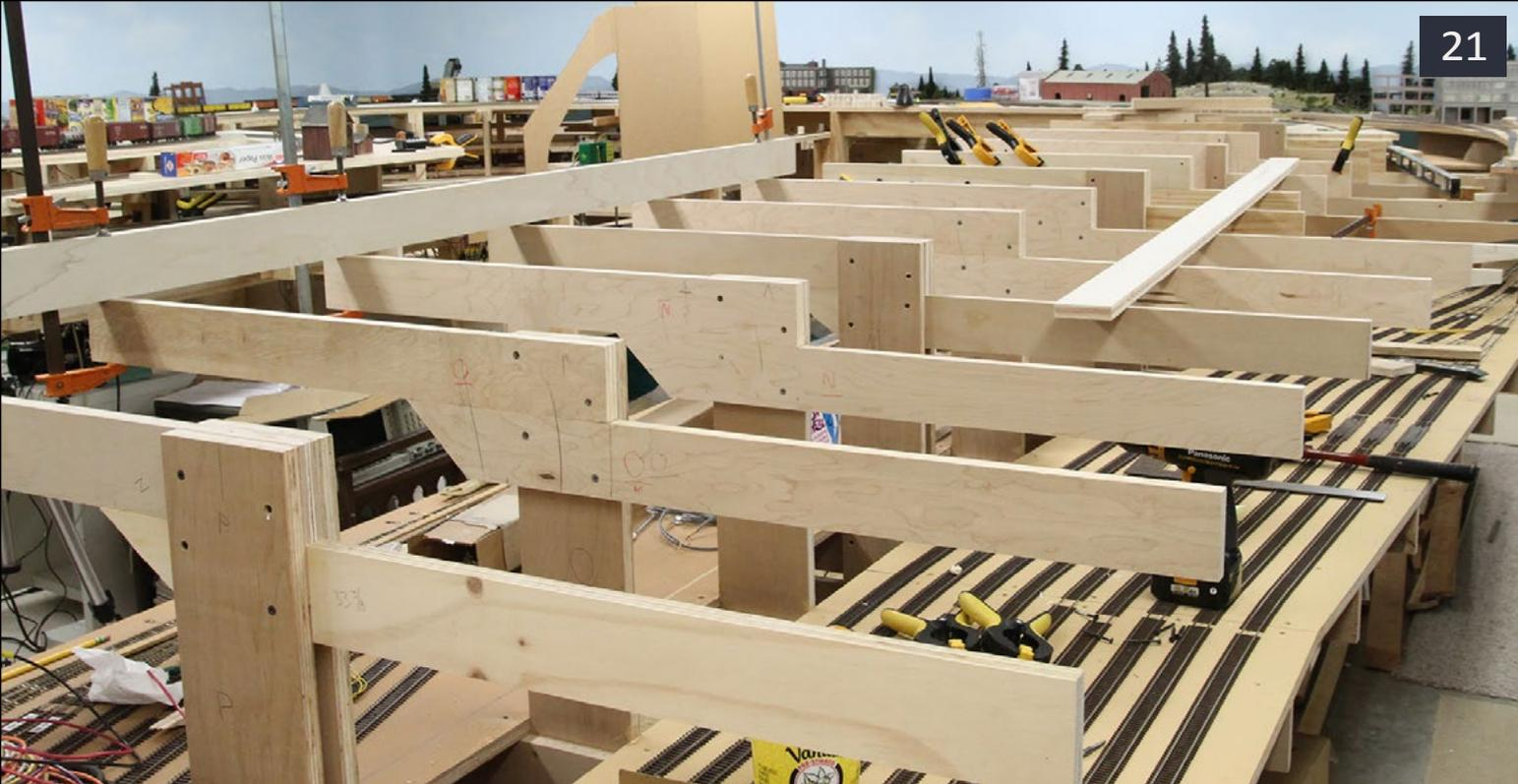
**21: These risers and joists will support the peninsula's upper deck. The joists are assembled using woodworking biscuits. The backdrop will attach to the "back" of the joists and risers. "Photo circa December, 2013"**
