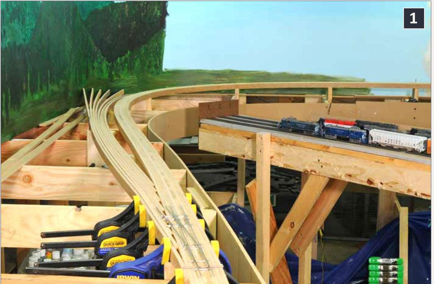
**1. Spline roadbed comes in many forms. These Masonite strips are laminated with carpenters glue, and can be built up as needed to locate switches. As long as attention is paid to maintaining a desired radius, splines can be formed into flowing transitions.**
