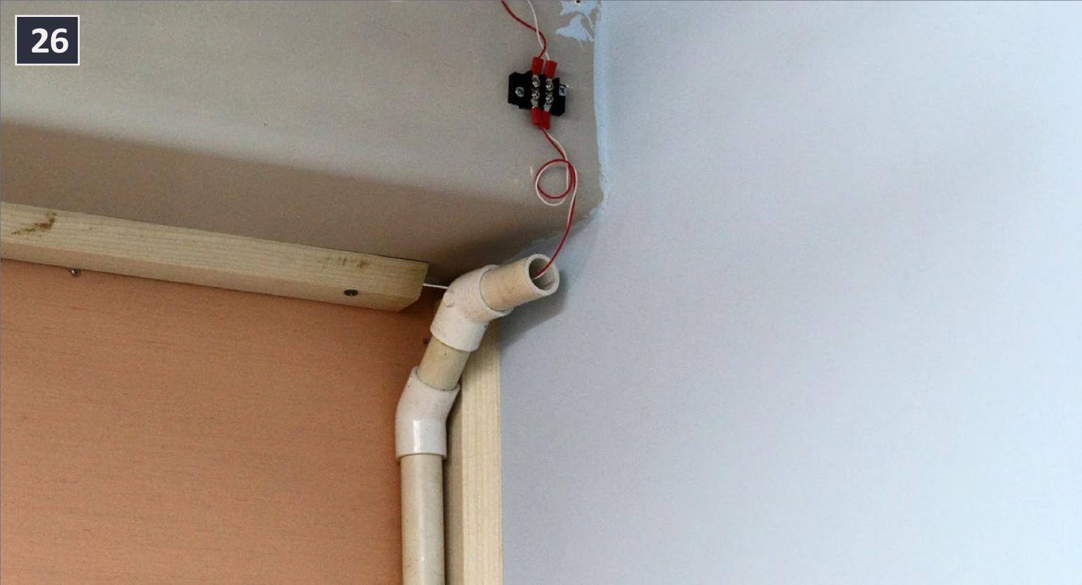
**26. A close-up view of the PVC conduit in the corner. This will be hidden behind coving and allows me to run future low voltage wiring from below the benchwork to the ceiling. The existing wiring is for the 4x fast clock.**
