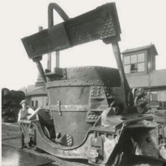
The cars were used to transport hot metal from the blast furnace to the Bessemer plant.
