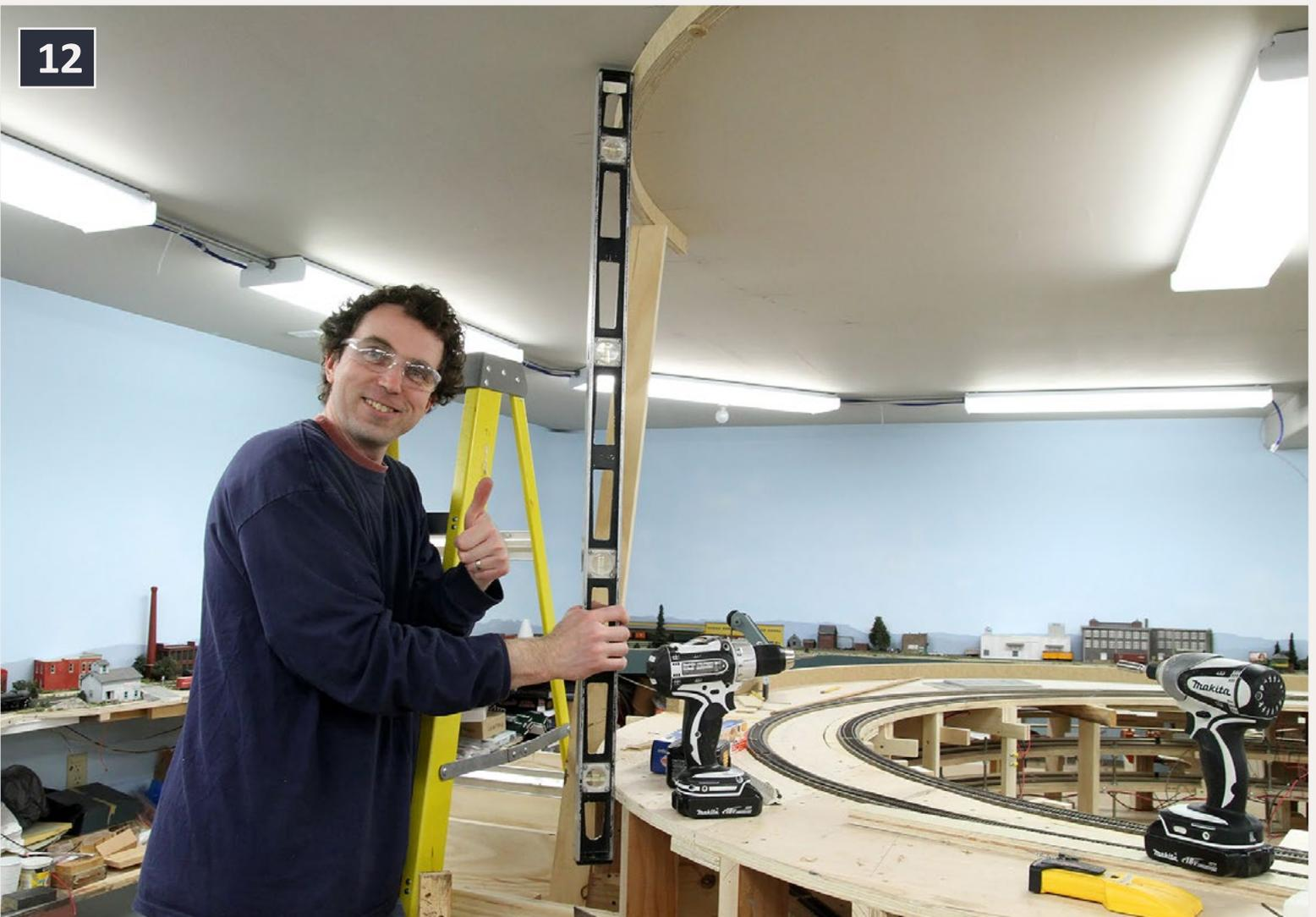
**12. We double-checked the ceiling cleat's alignment with the benchwork below. To our relief, it was spot on!**
