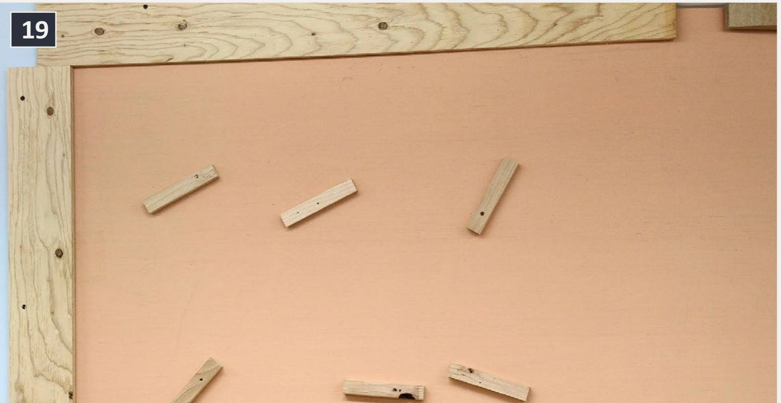
19. The temporary cleats (left and above) with the first piece of backdrop installed. The first 3' of the second layer has been glued in place behind this. I drove screws from the other side into the six scraps of wood to pinch the two layers of backdrop together for a stronger lamination.
