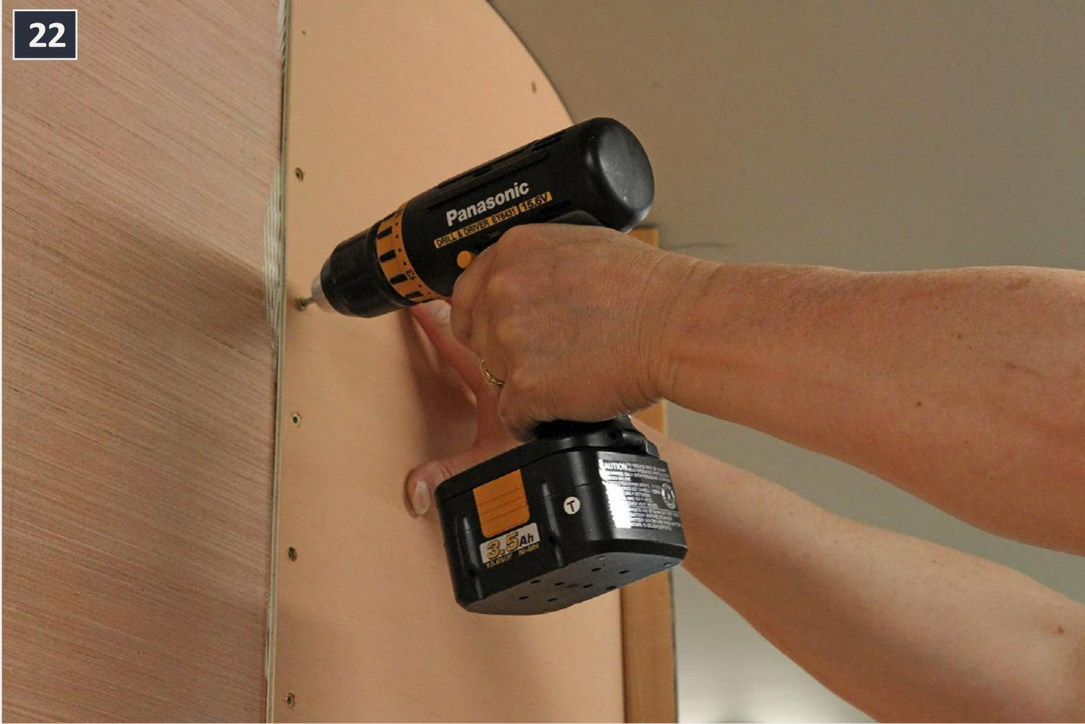
**22. There is a 2x2 temporary cleat on the far side of the backdrop. The row of screws I'm installing act like clamps (note the excess glue squeezing out) resulting in a strong joint. Once the glue sets, I'll remove the 2x2 and screws. The seam and the holes left by the screws will be filled with spackle. Clean up excess glue BEFORE it sets!**
