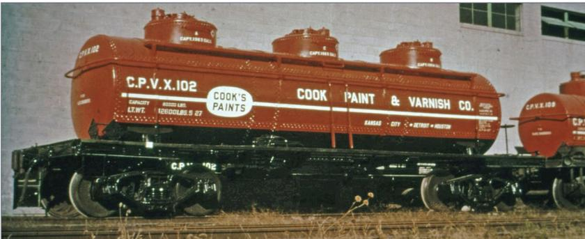
12. American Car & Foundry built this three- compartment 6,000 gallon tank car in May 1927 for the Cook Paint and Varnish Co. Note that, though freshly painted in the 1950s, this car still had its 5-27 reweigh date; tank cars were not required to be reweighed periodically, like other freight cars, because the shippers were charged by volume, not weight.
