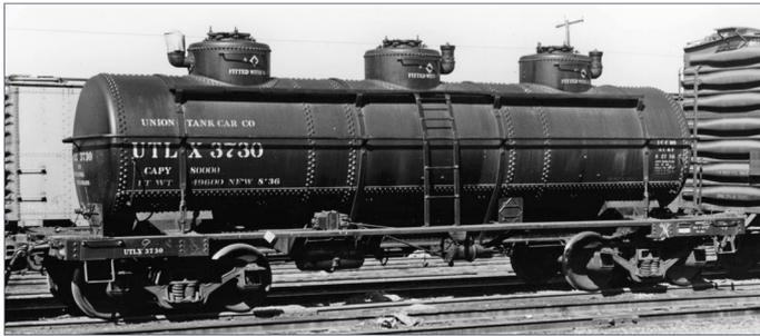
21. American Car and Foundry also built this 6,000 gallon three-compartment tank car for Union Tank Line in August
