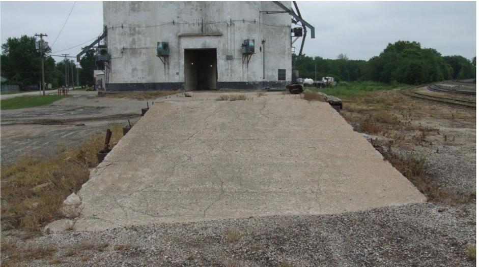
4. The ramp end of the loading dock, looking north. The interior of the entire structure was filled with sand and a concrete liner applied on top of the sand. May, 2008. Photo by Jared Harper
