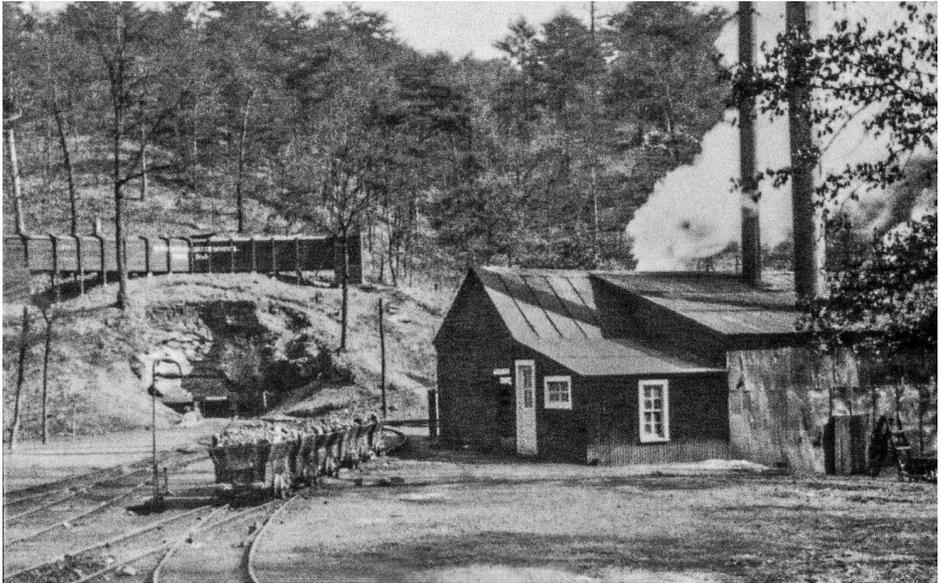
4. The Merkle Mine showing the trackage and the hoist house. The entrance can be seen to the left of the tiny mine cars. Phillip Griffith Collection
