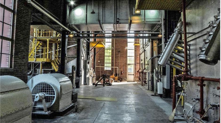
**2. Inside the boiler house today. Boilers 16 & 17 are on the left, and Boiler 18 on right. The tube in front of No. 18 delivered coal to a crusher which fed fuel into the boiler's firebox. The building is a lot cleaner than when it was in operation with the coal-fired boilers. Philip Griffith photo**
