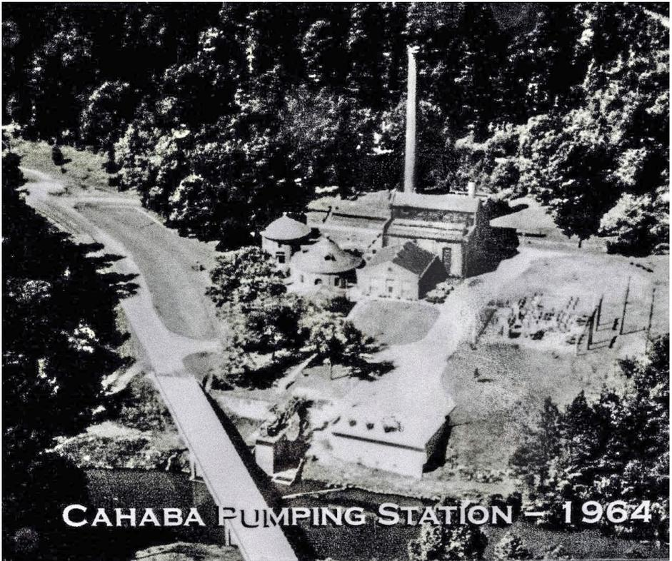
1. Aerial view of the Cahaba pumping station pumping station in 1964. This was after the pumps were converted to electrical operation, thus the power substation seen in the photograph, and 15 years after the railroad had been removed. Birmingham Water Works photo. Philip Griffith collection
