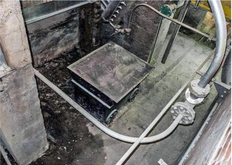
5. Ash track in the basement of boiler house. The car is an inoperable model and is there for show only. The car bears no resemblance to the real cars used in the basement. This must have been the dirtiest, nastiest job in the entire plant. Philip Griffith photo
