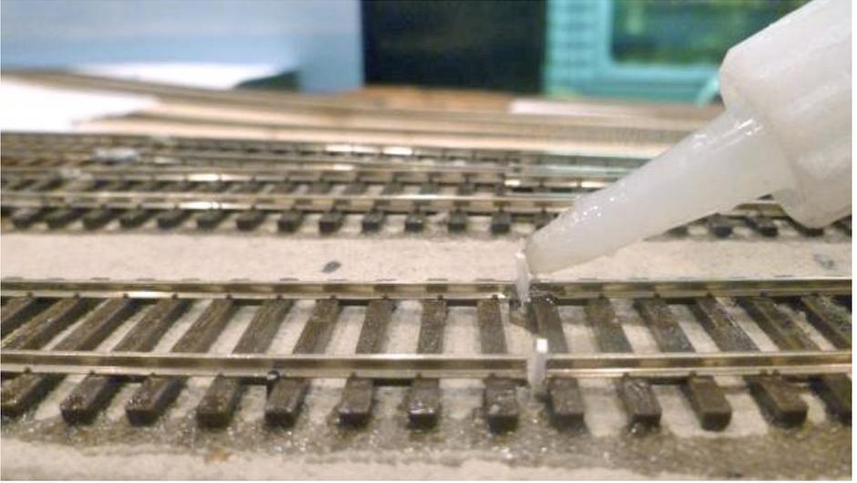
6. Gluing the styrene strip in place.
