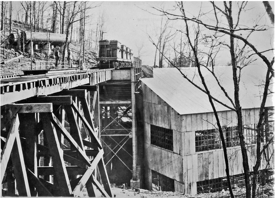
14. This “high line” apparently ran from the surface mine operation to the washer, which was under construction at the Vance Mine in the winter-spring of 1928-1929. *John Stewart Collection*
