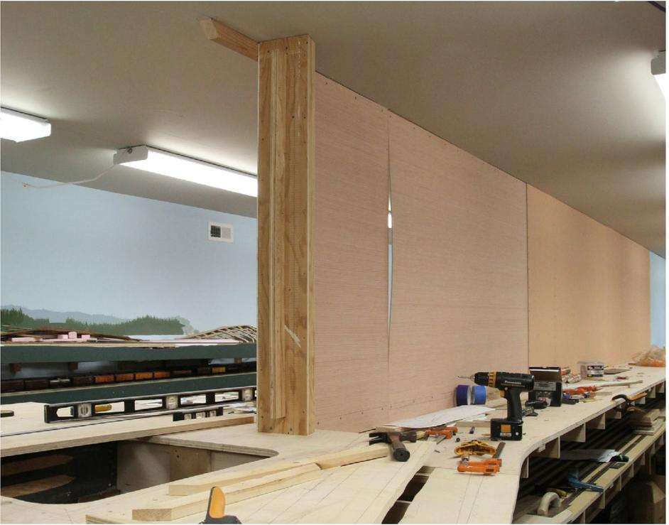
3. By late November, 2014 the peninsula benchwork was completed and it was time to get cracking on the back-drop. The two plywood laminations will separate about 24" from the end of the benchwork, and will be screwed to the bullnose mounting plate. This photo shows the first layer of plywood in place. Note the warpage of the plywood visible at the seam. Once the two layers are laminated, the bowing disappeared.
