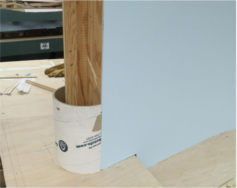
9. To tell the truth, I wasn't convinced we'd end up with a usable bullnose. You can see here that it did work – we placed one of the cut off ends of the bullnose against the mounting plate and it was less than 1/32" wider than the mounting plate on both sides. I can tell you this was a big relief!
