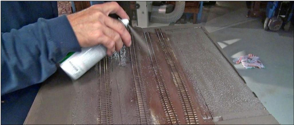
16. I laid two siding tracks to serve the building. This track was glued down with Liquid Nails, then painted with Rustoleum Camouflage paint to give the entire area a dull, even tone.
