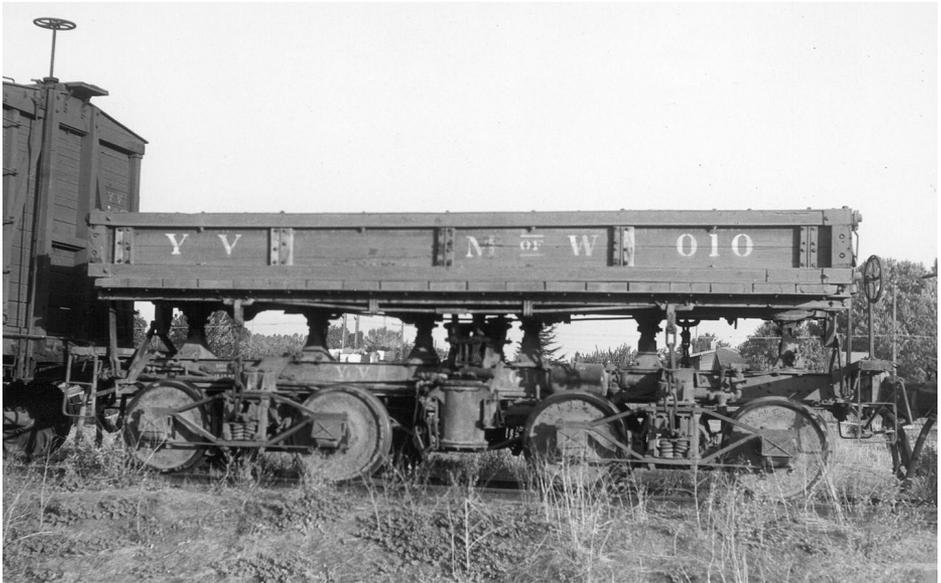
21. At first glance, scratchbuilding a model of this side dump car appears to be nearly impossible given the complex design of the frame, the pedestals which allow the bed to be tipped to either side, the U-shaped supports for the bed, and the complex rods and levers which actually tip the bed. However, with experience and by working methodically, it is completely possible.
