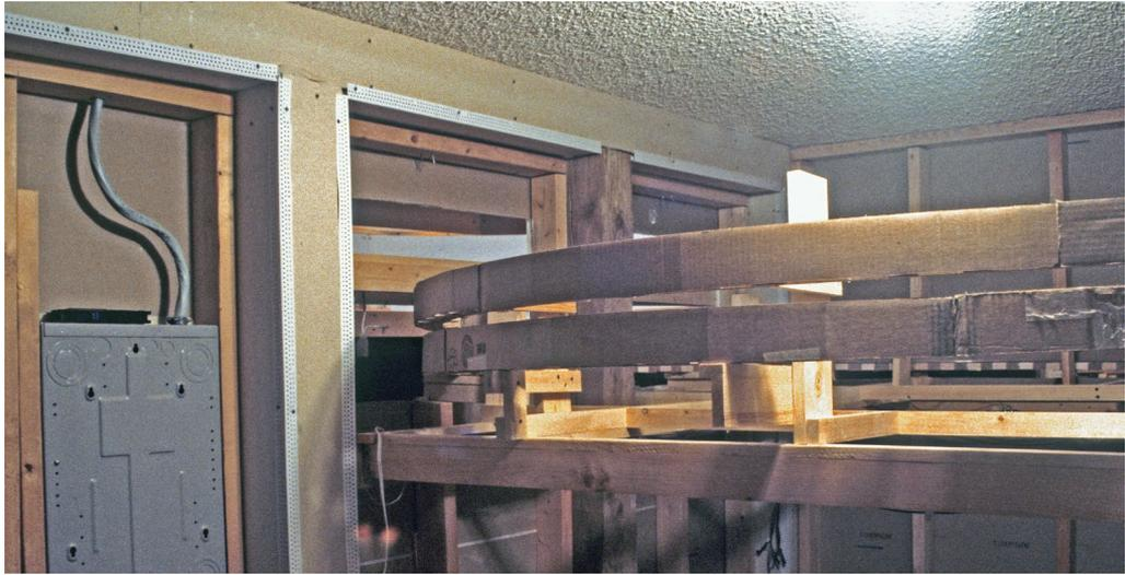
16. Here's the 40-inch radius helix in my workshop that replaced the 24-inch radius helix. This much larger helix with a 1.75 percent grade operates far better than the other helix – the difference is like night and day. The cardboard along the outside protects derailing equipment from heading toward the floor, although derailments in the helix have been quite rare.
