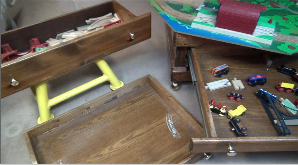
12. I built three drawers into the base to hold track and trains. Wheels on the base make for easy vacuuming under the table.
