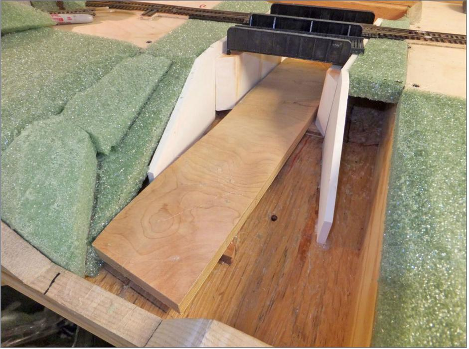
80. A new piece of plywood is installed to the proper height and will form the stream bed base. I don't like to use foam under Enviro-Tex as I've heard it can out-gas and cause bubbles. True or not, why take the chance?
