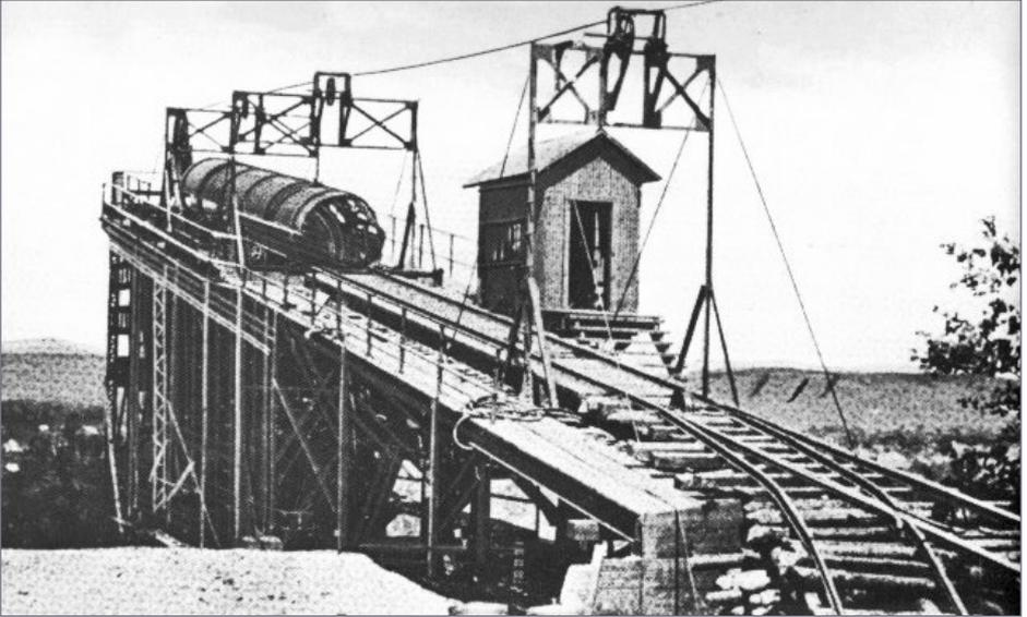
7. Woodward Iron tippel, either No.1 or No.2. Note the overhead cable sheaves that pulled the cars to the top of the incline for dumping. Photo from *Mine, Mill and Microchip, a chronicle of Alabama enterprise*, Wayne Flynt, Windsor Publications, 1987.
