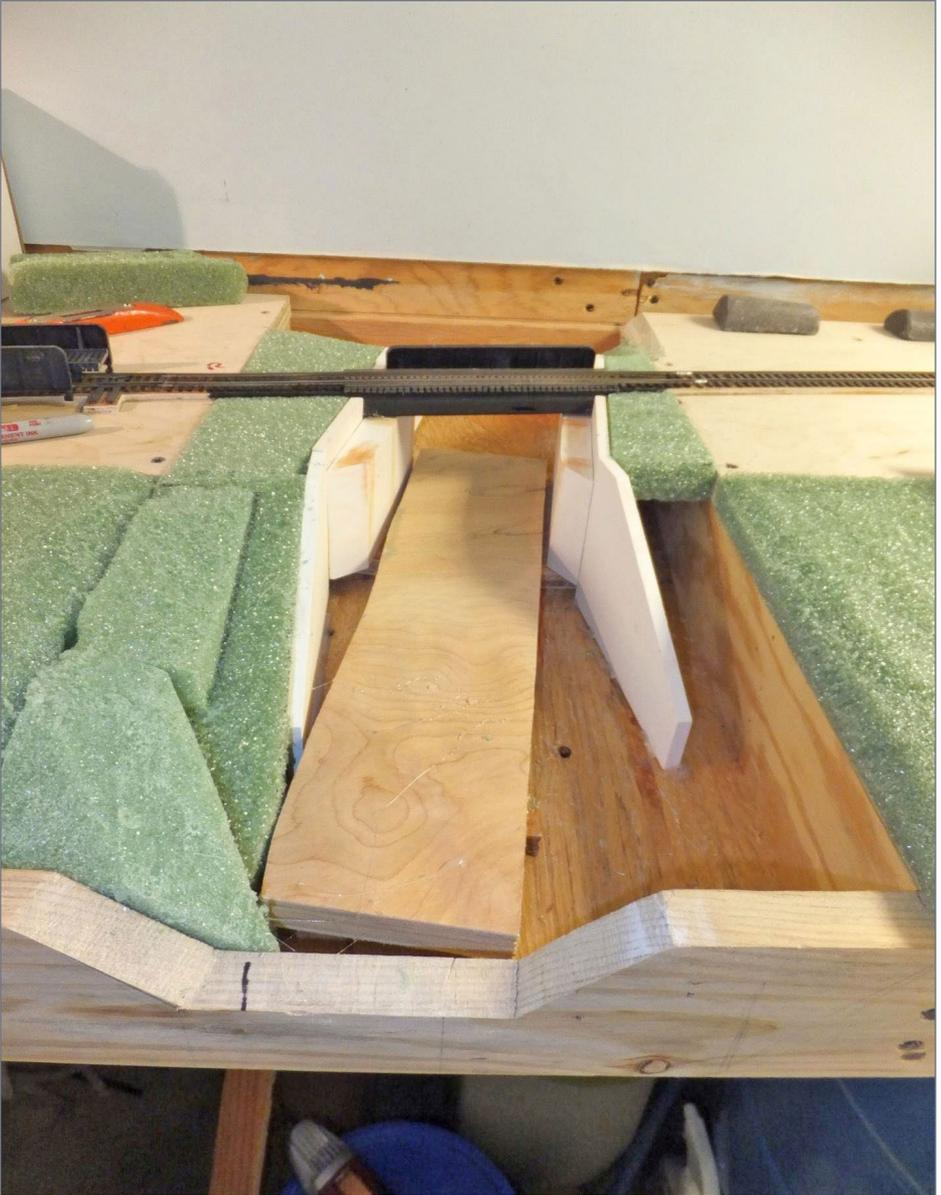
79. With the stream bed properly defined, it is now possible to cut the front layout joist and to fill in the embankments with foam.
