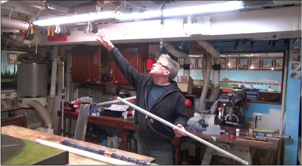
18. I tested a new type of LED shop light fixture bulbs. These are totally new and use only 17 watts each. They cost around 22 dollars per bulb but I'll bet that price will come down over the next year. Here you see me installing the bulbs for our overview. The light above my head is the LED bulb. The light on the left is a regular fluorescent. The LEDs seem brighter than the regular bulbs and use less than half of the electricity.
