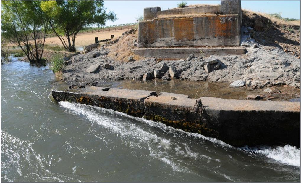
5. A current day view looking west shows an abutment and the pier for one of the trestle bents. The holes in the far side of the pier show that it was poured around the original driven-pile bent. That bent would have been sawed off after the new bent was in place.
