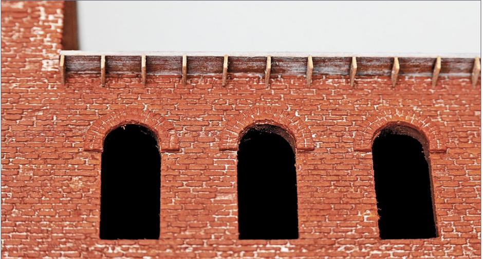
1-2. The rafter tails on the 1900 building [1] are boxed in with wood. The tails on the 1880 building [2] pass through the brick wall. The rafter tails are short 2x8 segments bonded to the overhang.
