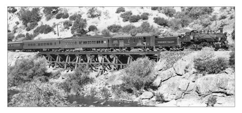
5. Here the passenger train crosses Bridge 64A at Fox Creek. Note how some of the trestle piers are "stepped" after the original mud sills were replaced with concrete piers.
