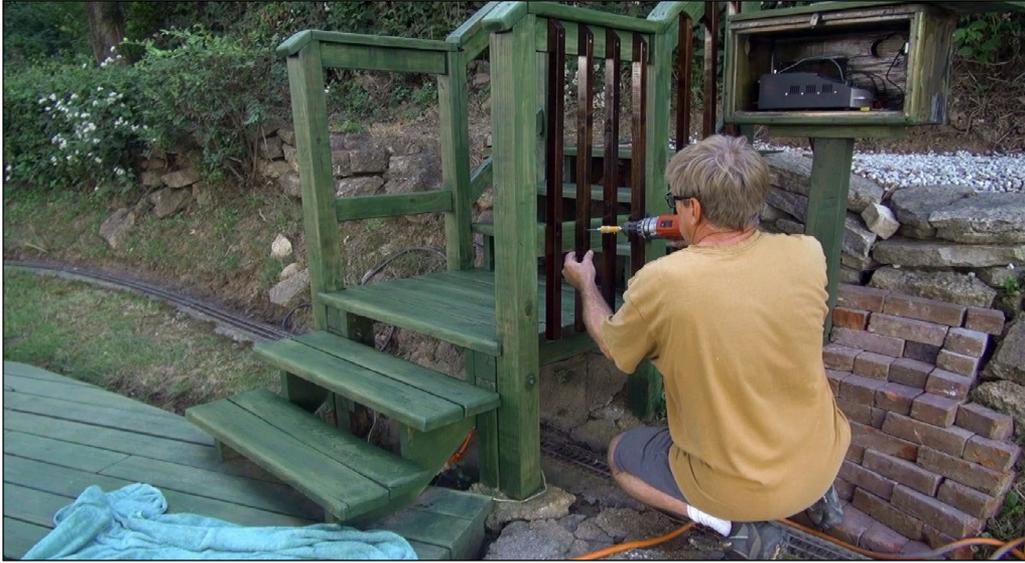
8. I applied a fresh coat of semi-transparent green stain to the deck. I stained the stair trim pieces with brown stain, and reattached accent wood to the deck.
