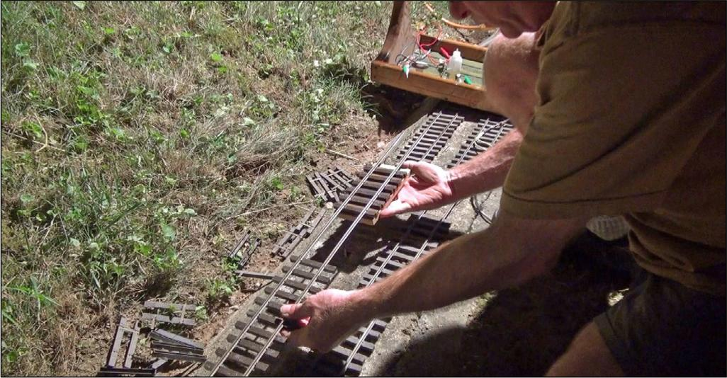
2. This process included replacing some damaged plastic ties with fresh new ones. With the help of a handmade wooden jig, the ties slide on to the rails.
