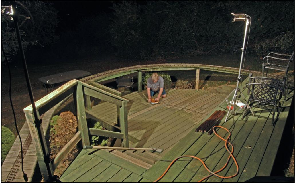
7. I sanded the train deck where the dogbone layout loops back – sanded it down to the bare wood with a six-inch orbital sander and 60 grit paper.
