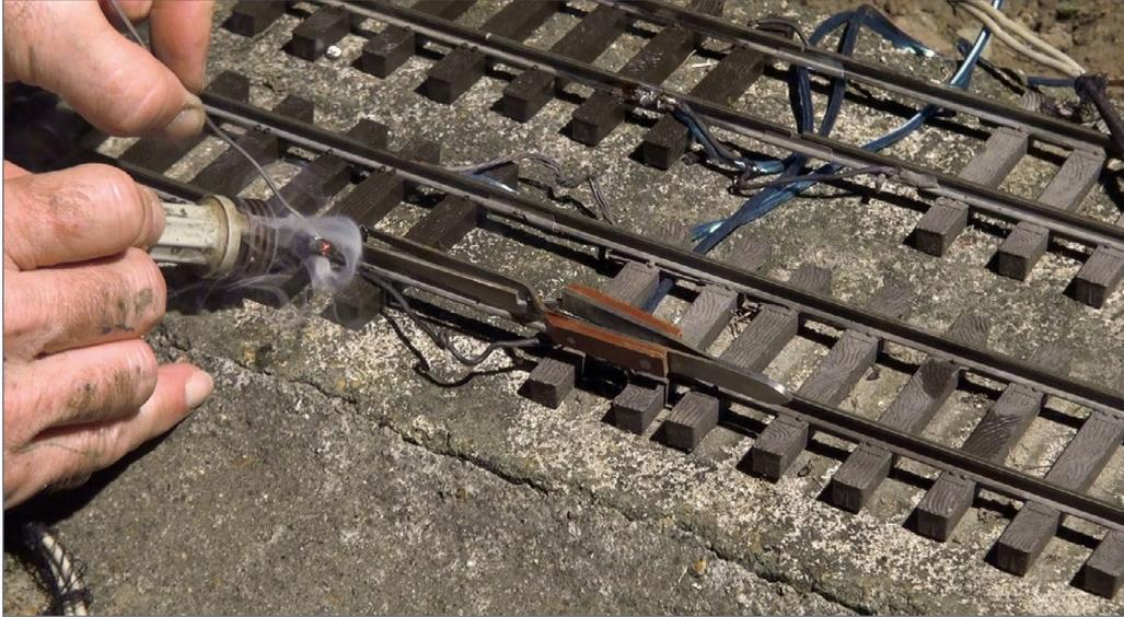
3. I added new power feed wires in eight spots on the 400-foot main line by using a resistance soldering rig to heat the large rail fast and minimize damage to the plastic ties.
