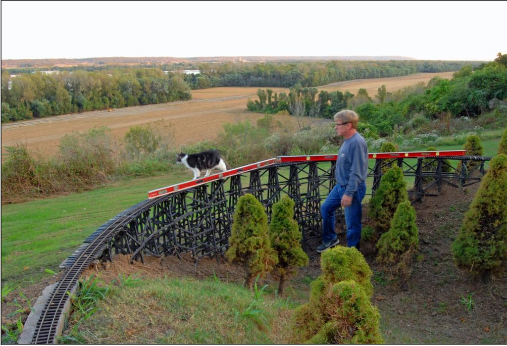
6. The next day, using an eight-foot and a six-foot level, I rechecked my work to make sure the trestle was level end-to-end and level from side to side. The train needs to run perfectly here to avoid a four-foot crash to the ground. Wind is the worst problem here. Anything over 14 mph will blow a train off domino-style. I have seen it happen many times.
