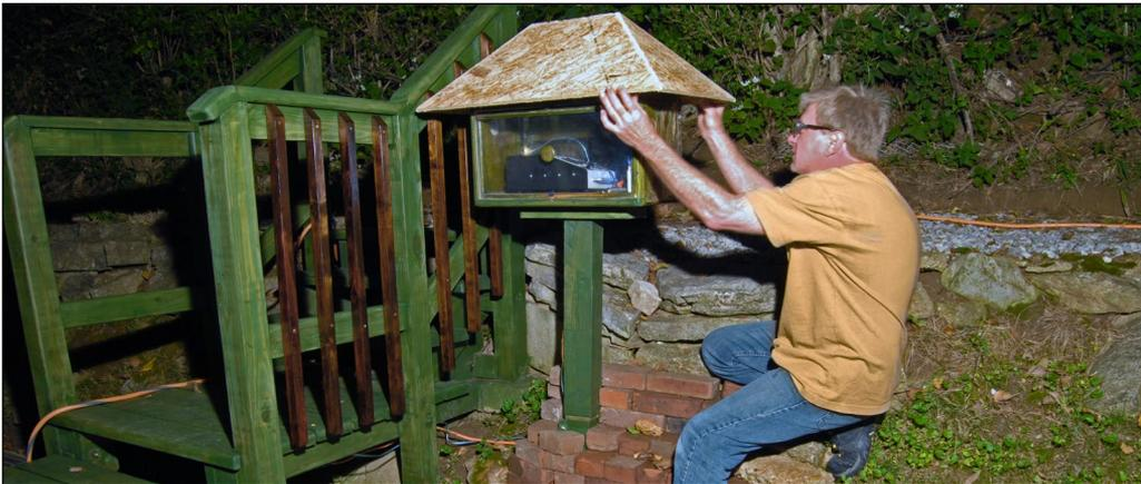
9. I built a waterproof box of wood on a pole, with a hip roof, to house the electronics and power supply. This was hidden under the deck before but I erected it on a pole for better radio reception with the hand-held radio controller.
