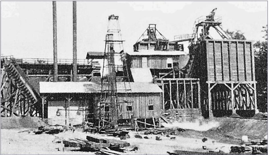
4. Twin Seam (Central Coal and Iron) tipple and washer Number 1. *Department of the Interior Bulletin 400 dated 1910*
