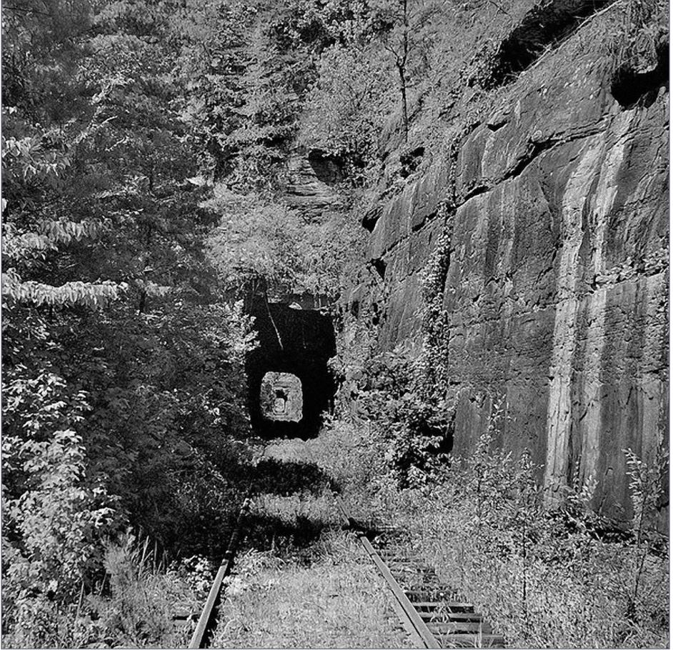
28. View is west into fourth tunnel up Daniel Creek from the Black Warrior River. The third tunnel is seen in the distance through tunnel 4 and across two trestles. Distance to the distant second tunnel portal is about 1500 feet. Tunnel 4 is 300 feet in length, then a 190 foot trestle, then through a cut and across a 225-foot trestle to 500-foot tunnel 3.
