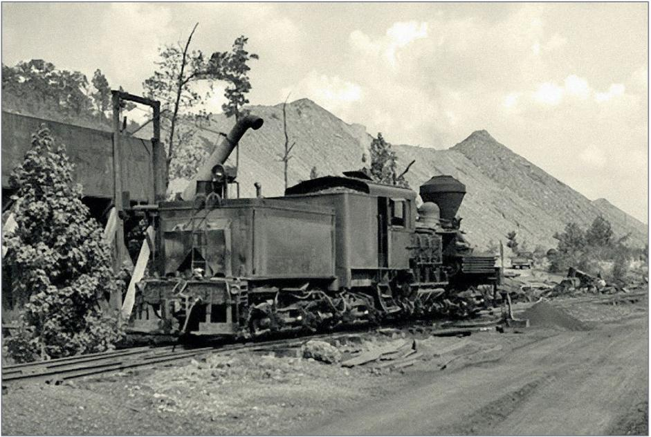
7. Shay No. 5 taking on water at the Kellerman water tank. The tank is a converted tender with a spout added.
