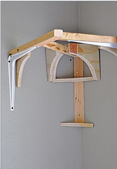
8. I added the brackets and extensions adjacent to the corner pieces, plus some additional cove pieces so there is plenty of material to screw the Masonite into.
