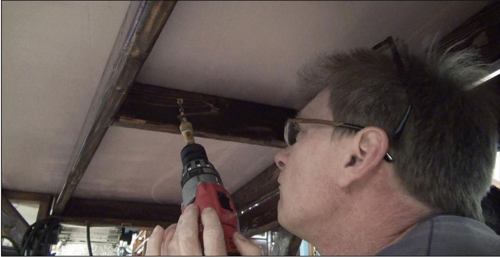
16. To prevent the foam from sliding on top of the bench work when pushed or bumped, I drill countersunk holes in to the bottom of the wood, and drill three-inch screws up into the foam. This holds it firm yet makes it easy to detach quickly to move the layout outside for photos or video when needed.
