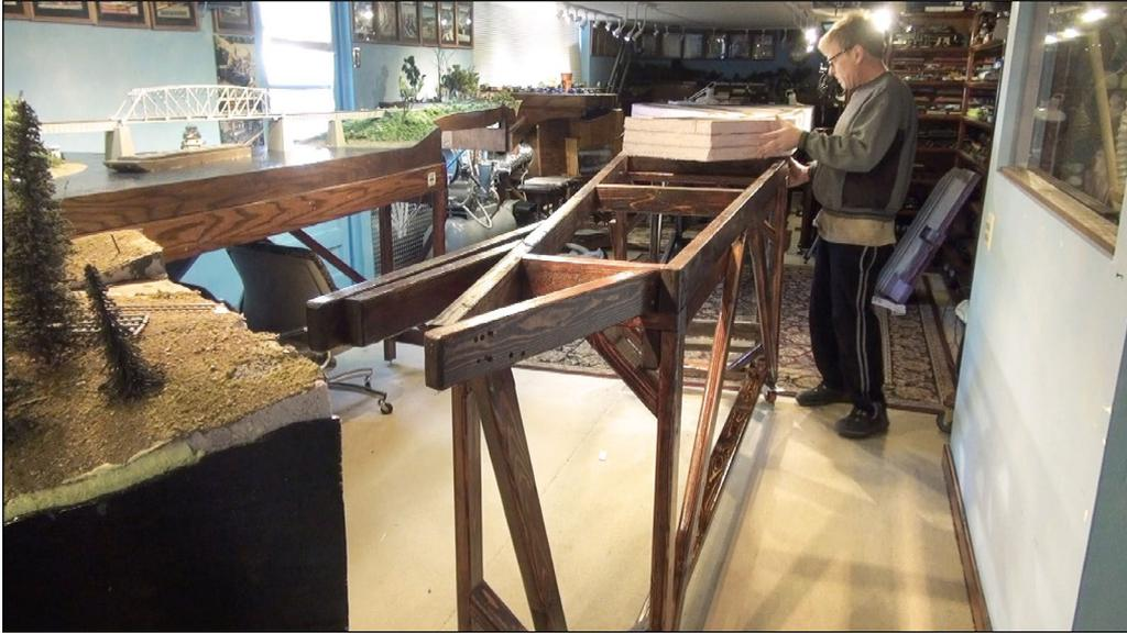
14. Now it is time to put all the pieces together. I roll the benchwork into position close to the bridge module that will connect with the sawmill diorama. If my measurements are correct, the rail height will match perfectly on both scenes as they go together. I slide the sawmill diorama on top of the smooth benchwork. I carefully position the foam even and square to the benchwork, matching marks I drew on the foam underneath to ensure an exact placement on top of the benchwork.
