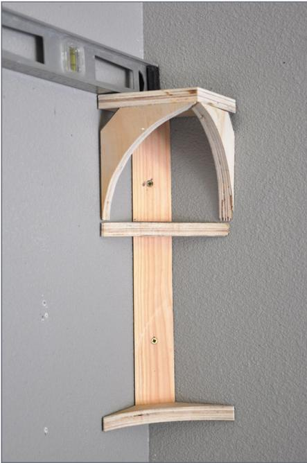
7. The corners were installed first, then I leveled the top of the backdrop using them as my height guide. The spine of the corner pieces are sections of 2x4 that I ripped at a 45° angle and attached to two of the curved pieces for the cove.
