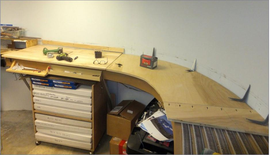
18. The pre-cut sections of new sub-roadbed are staged for installation. The straight sections could easily be attached to the wall cleats and I used shelf brackets for the curved section.
