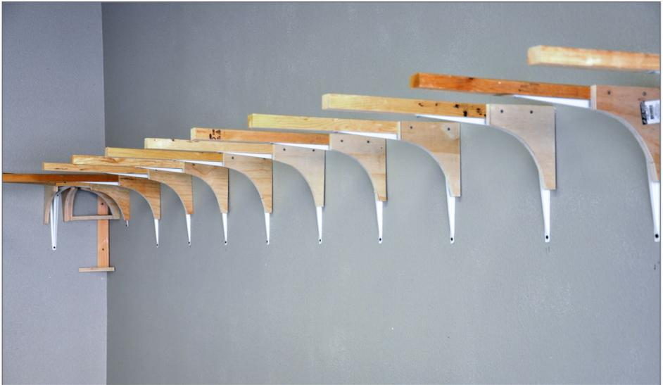
9. The shelf brackets have been installed, and 2x2 furring strips and the cove pieces have been added. Now it's time for the Masonite.
