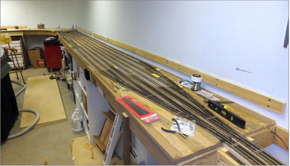
17. I created an entirely new yard ladder for staging, removing the old Custom Trax turnouts but leaving the track and using new Pecos. You can also see the cleat for the new staging yard on the wall.
