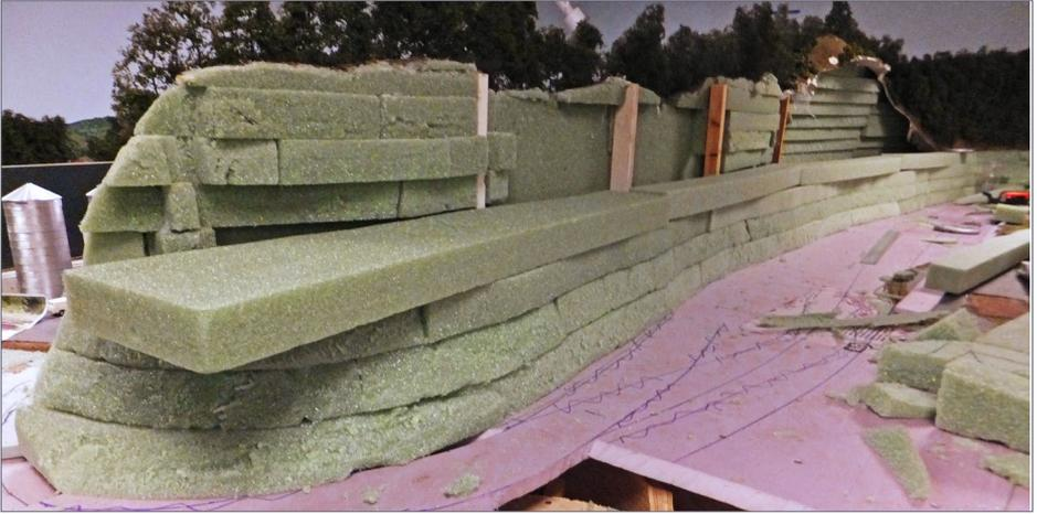
10. For each successive layer it was just a matter of placing pieces, tracing from below with a Sharpie pen, cutting them out on the band saw, and angling each one back by eye.
