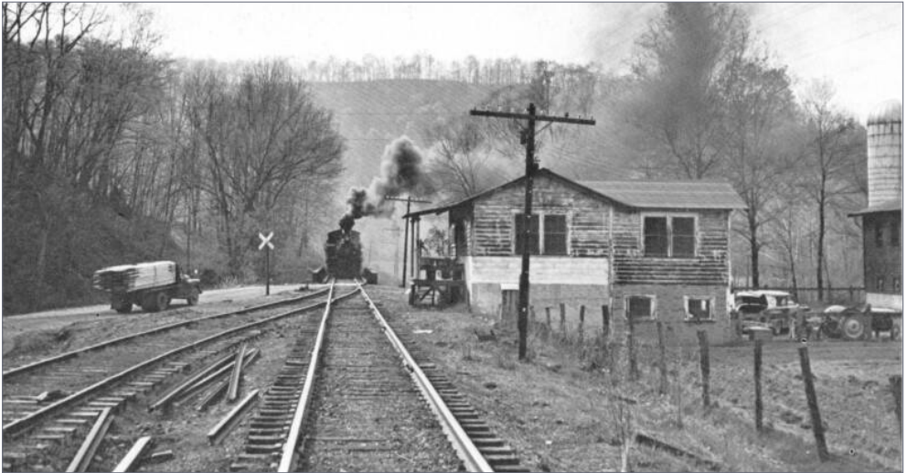
19. Cressmont Dairy end view.
