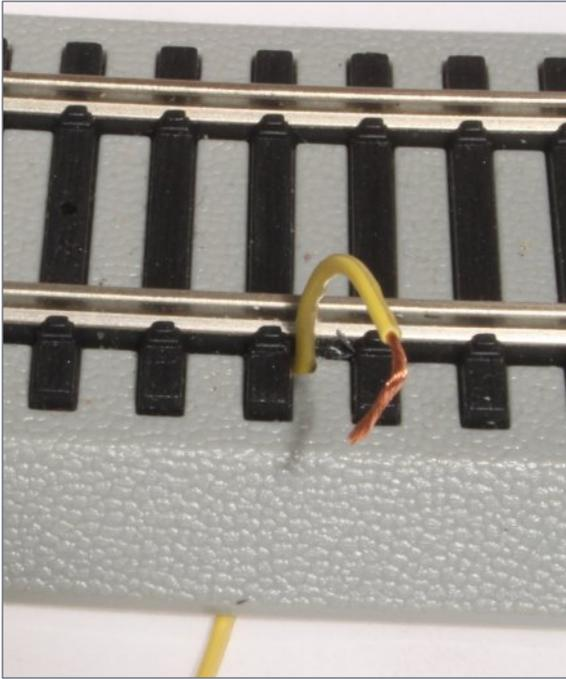
14. Slip the wire up through the track from the bottom. Strip 1/4-inch of insulation, twist the strands tightly and bend them over 90 degrees. Scrape the web of the rail clean with a jeweler's file.
